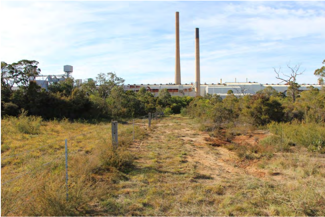
Plate 1 View across part of site Hydro-AS26-14, looking east
