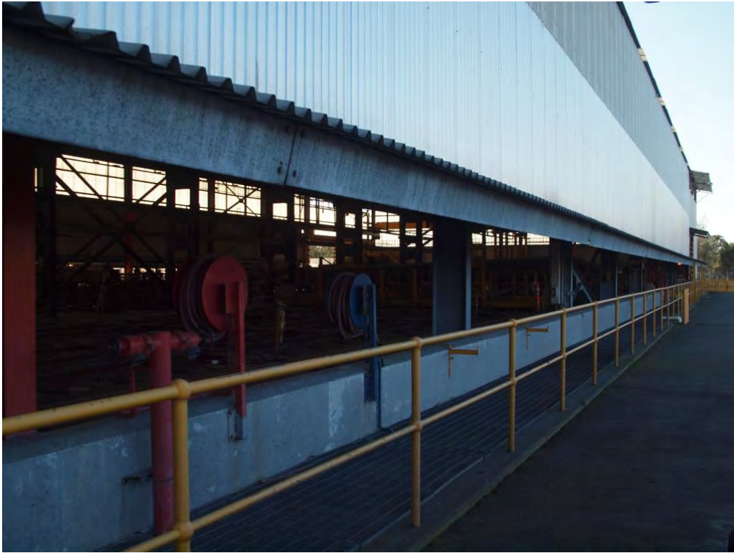
Plate 5 Carbon Plant – exterior southern wall
