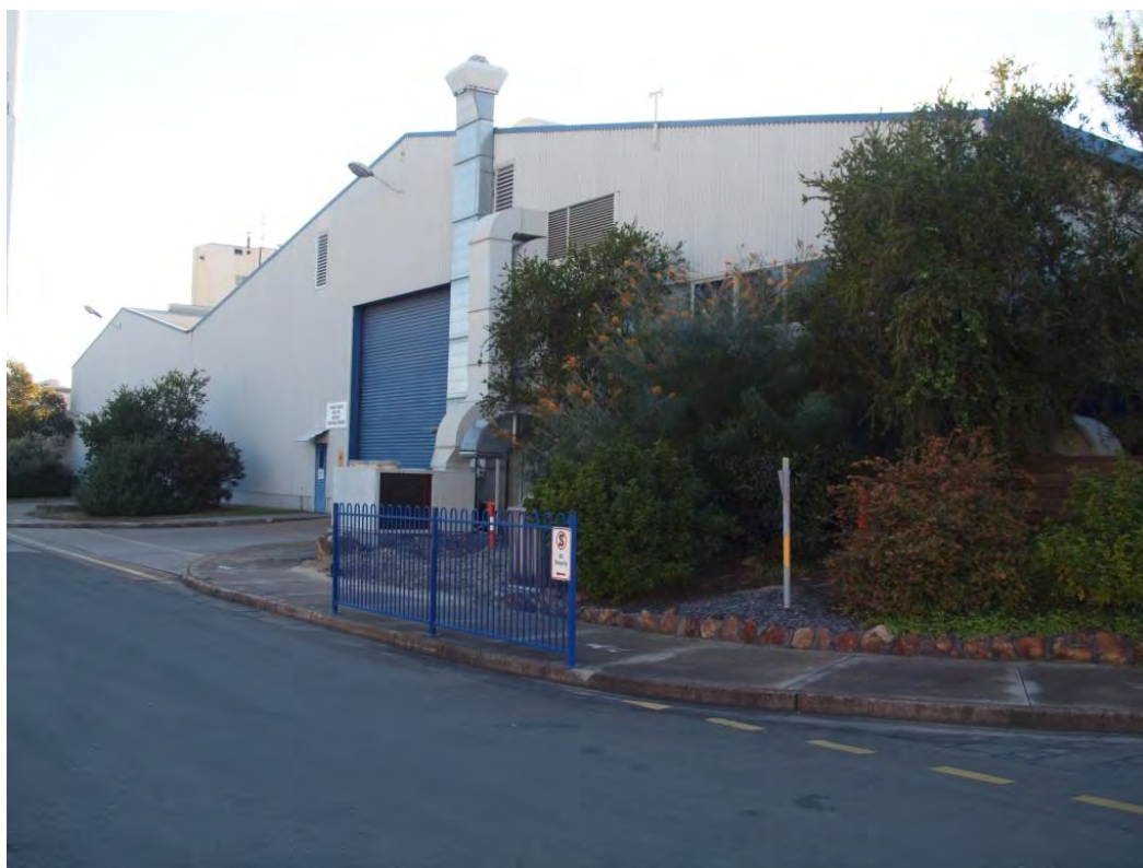
Plate 24 Ancillary buildings – Engineering
