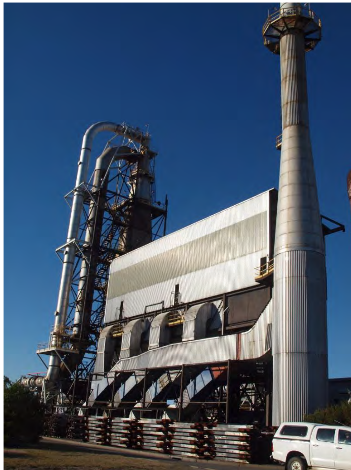
Plate 8 Looking south east to Scrubbing Plant
