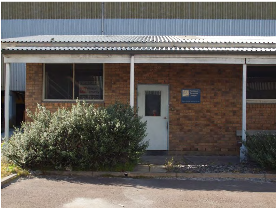
Plate 26 Ancillary building – Potroom Process Centre
