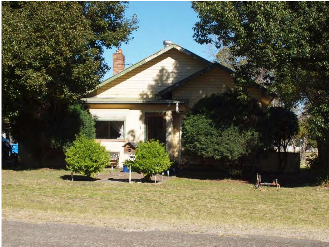
Plate 38 Weston Soldier Settlement: 1 Macleod Road - original house
