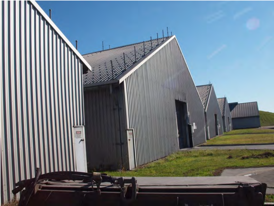
Plate 27 Ancillary building - Potline storage sheds
