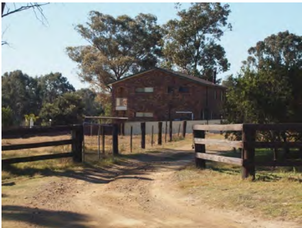
Plate 40 Weston Soldier Settlement – example of later housing
