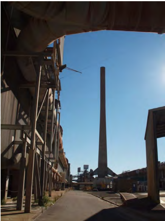
Plate 20 Looking north to chimney
