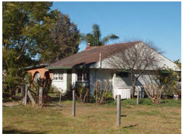
Plate 41 Weston Soldier Settlement – example of later housing
