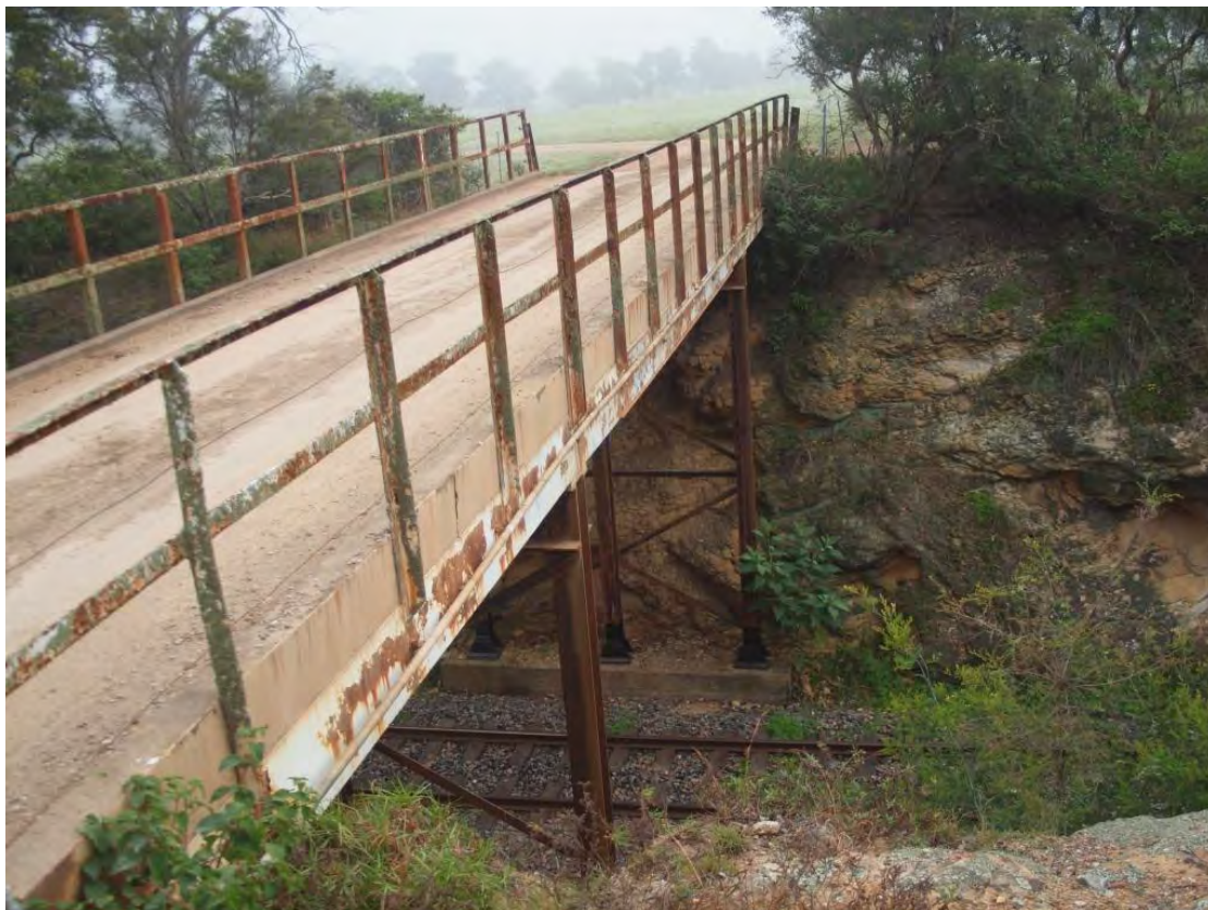
Plate 29 South Maitland Railway bridge
