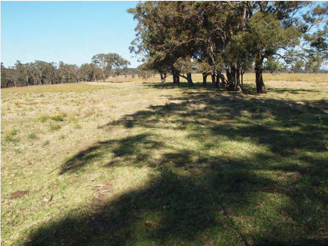
Plate 32 Stanford Railway – looking south east along embankment
